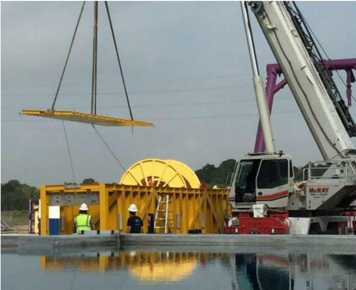
*Figure 18, Lid of storage tank being attached for pressure test.*
